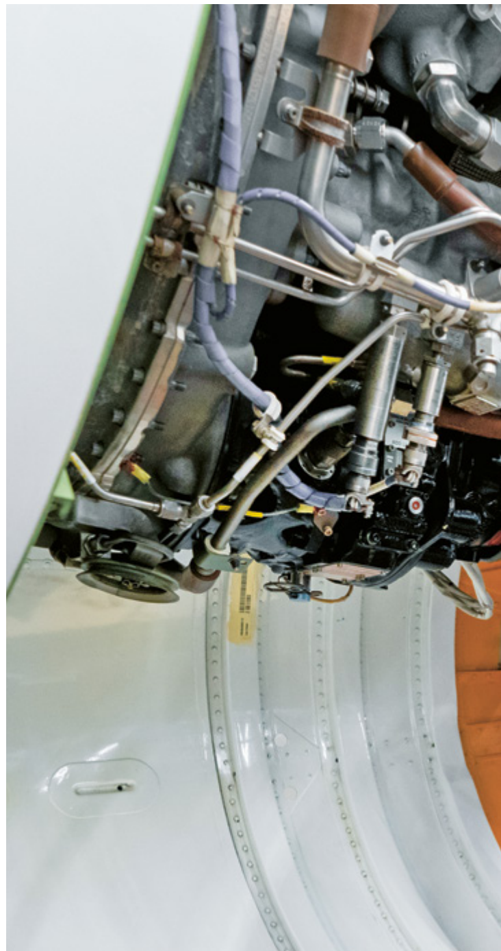
Checking, repairing and maintaining according to the specifications: every six months, the jet mechanics devote themselves to the engine of the ambulance jet.
